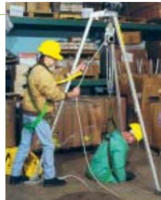
A secondary fall arrest system is recommended.
